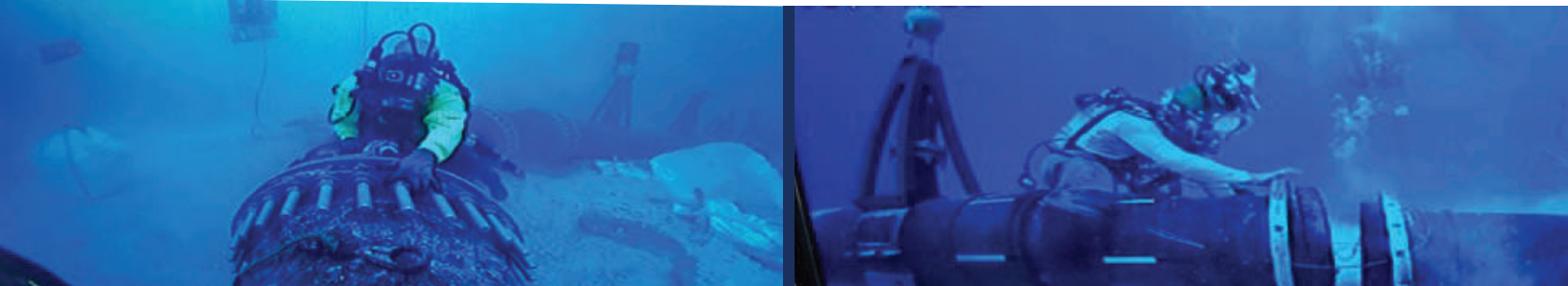
Outfall Effluent Diffuser Installation Project's Underwater Shots: These pictures were taken during the installation of diffuser pipes below sea level as part of the Northern District Treatment Plant Upgrades. The project successfully installed a critical environmental upgrade to the existing ocean outfall pipeline designed to protect the coral reef and marine fisheries along Tanguisson Beach. As a result, the project contractor received a national award for "best environmental enhancement project." Read the article using the following link: Contractor for Guam wastewater outfall diffuser project receives national award | Guam Business | postguam.com
