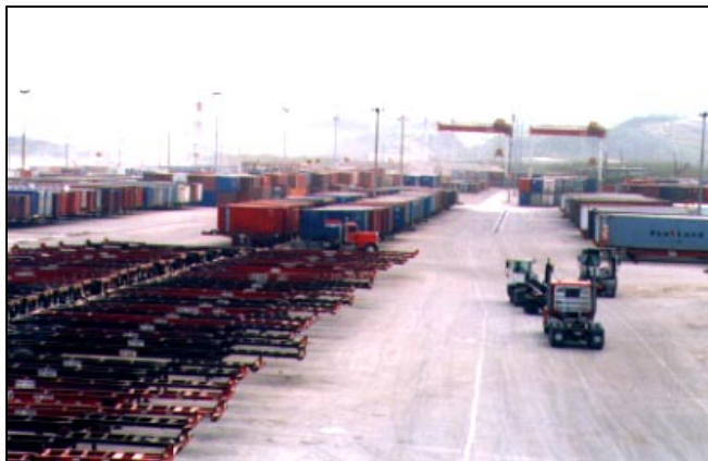
Image 2: Container yard at the Port Authority of Guam.
